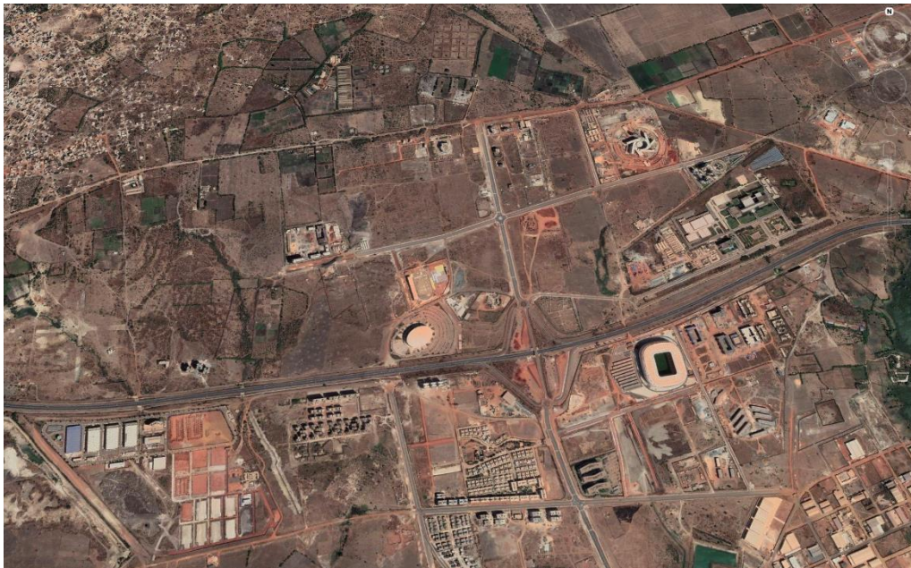
Bird's eye view of the construction work in Diamniadio. The construction process is slow and fragmented. © 2022 Maxar Technologies
